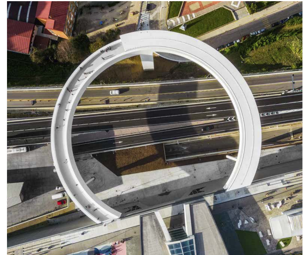
Next to these lines: the structure makes it possible to overcome the physical barrier posed by the highway and a 40-meter drop in elevation. The Butech façade department developed, fabricated, and installed the project's Krion® Lux 1100 vestiments, with an industrialized system that provides higher quality finishes with shorter execution times. On the previous page, at the bottom: a section of the walkway is covered to protect pedestrians from inclement weather. The entrance to the upper part of the building is spacious and open-plan to facilitate accessibility. Below: view of the tower and curved walkways from below, where the elevator access is located.
